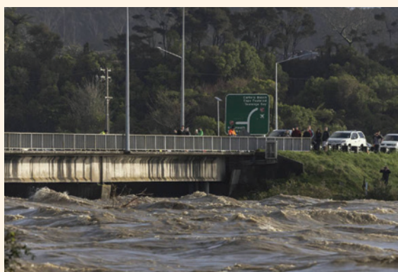
Buller River Bridge – Westport (Source: C McLachlan)
